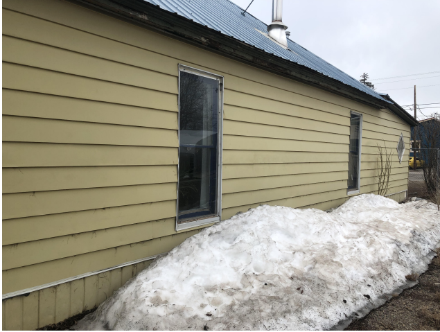
Figure 7: Possible ccASHP location on north side of house
